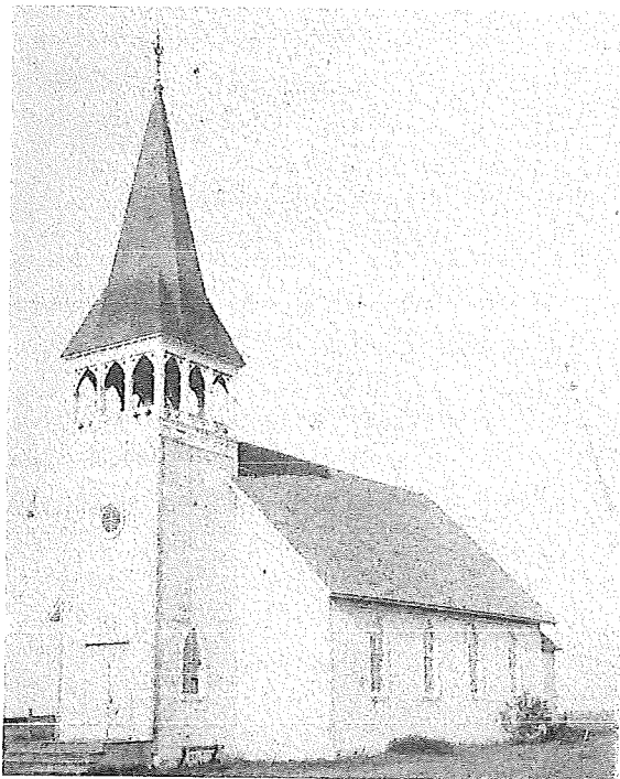
The original G.A. Lutheran Church building.
